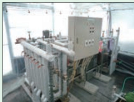
Geothermal heat pumps installed in the air house of Hokkaido Niseko High School
