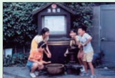
Rojison, rainwater storage tank in the city
